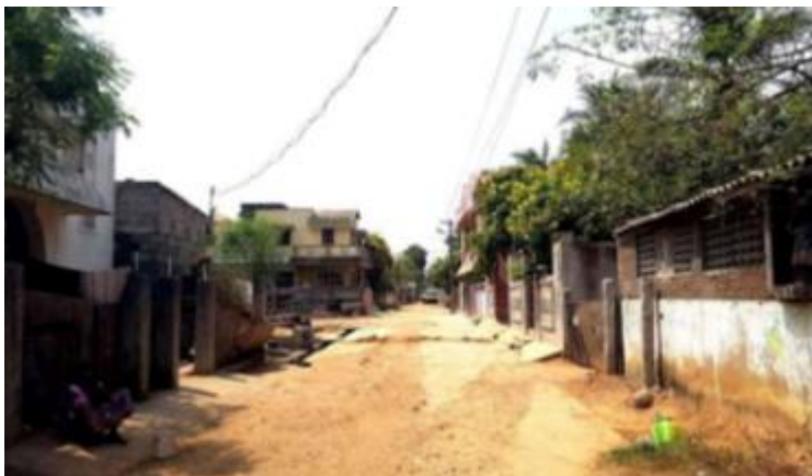
Figure 19: Lack of basic services in Katchipattu
